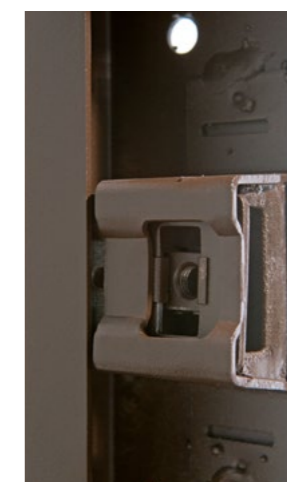
Detail of frame-preframe regulation
