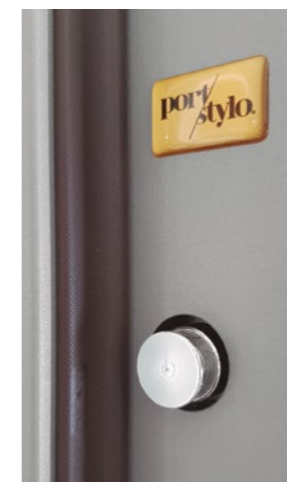
Governor bolt and acoustic seal
